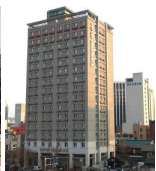
CO-OP RESIDENCE EULJIRO
