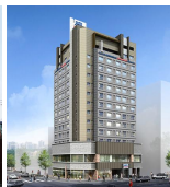
CO-OP RESIDENCE DUNSAN HOTEL
