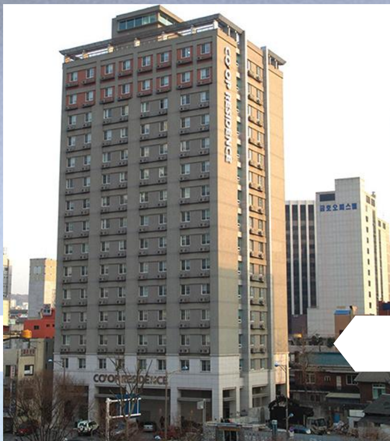
CO-OP RESIDENCE EULJIRO
